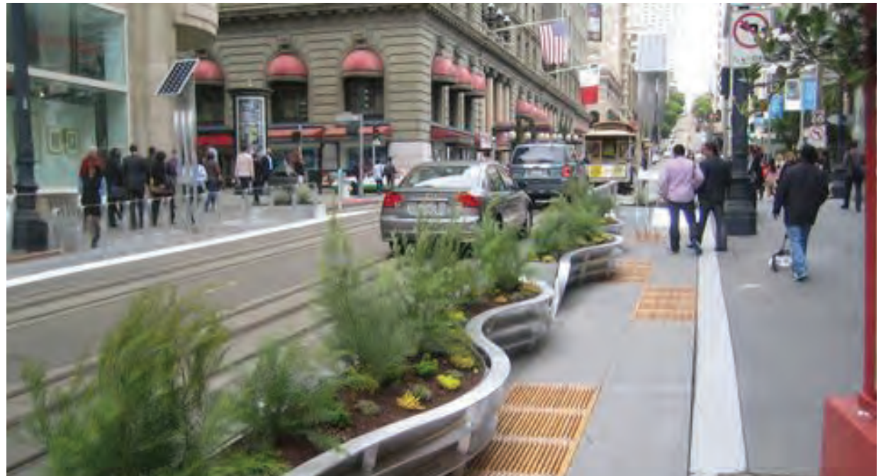
Figure 24: Precedent examples of interim streetscape enhancements that create space for desired activities
