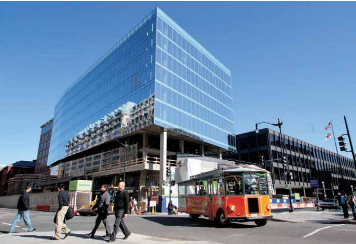
Skanska USA Commercial Development began construction on this 10-story building at 733 10th Street in the summer; the delivery date is in 2011.
