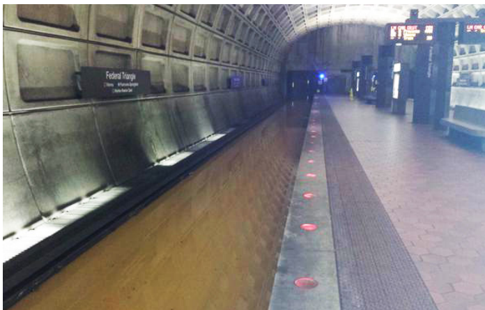
On Dec. 14, 2014, a water main break at 12th and F Streets, NW flooded several stations, including Federal Triangle, during rush hour. (Photo: WMATA)
