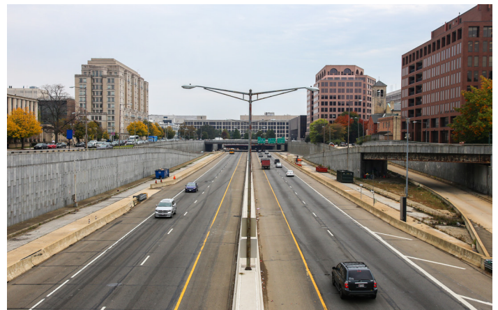
Infrastructure construction has begun on Capitol Crossing, a $1.3 billion project that will deck over the I-395 freeway, reconnecting the East End of Downtown to Capitol Hill.
